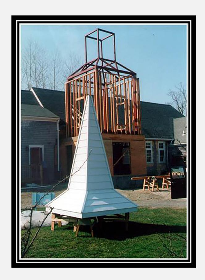
The major exterior work involved construction of the narthex and bell tower/steeple. The steeple was fully assembled before being raised over the narthex. The sea bass weather vane was its crowning touch.
